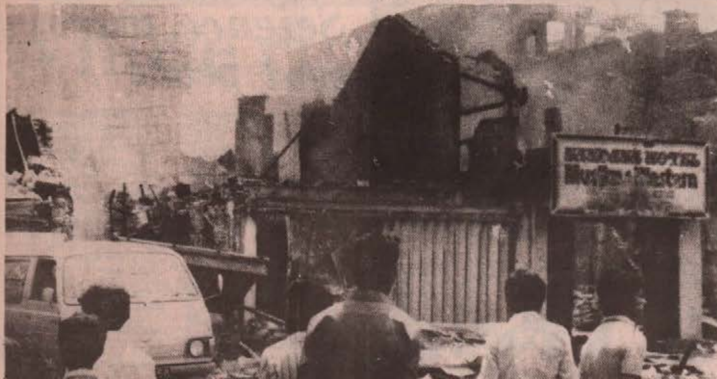
Tamil building gutted in 1983 pogroms
